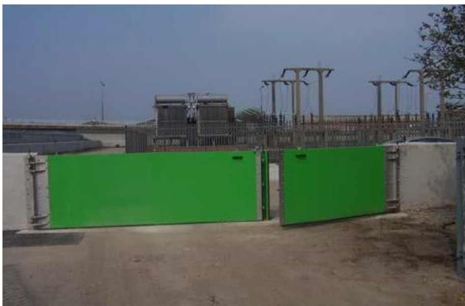
Figure 6.6: Flood protection gates (ENA ETR138 Annex 1)
